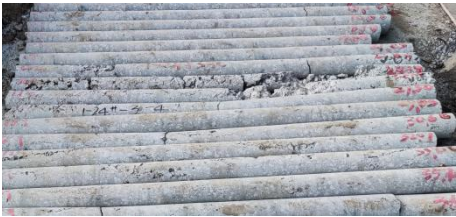
(a) 1-24#桩 3#孔芯样
